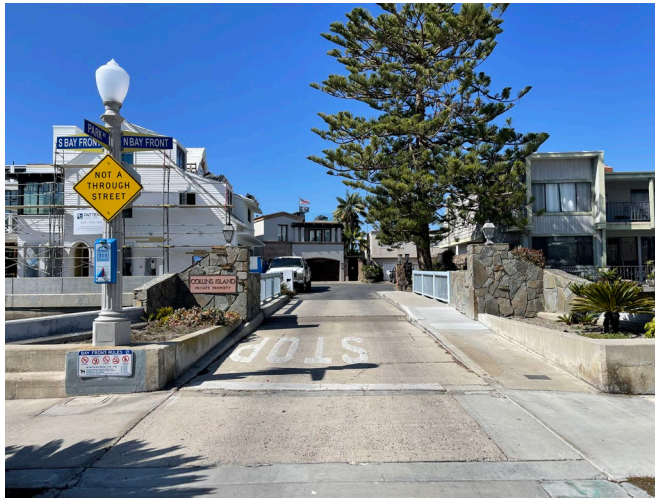
View looking at existing bridge, towards Collins Island.
